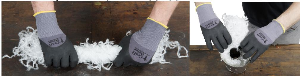
Push in more packing material with a suitable tool without pressing it too heavily. In doing so, pack the entire weighed packing material evenly up to the top in the silencer.
